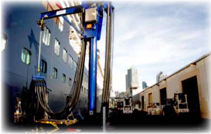
Cruise ship connected to the Port of San Diego shore power system.
