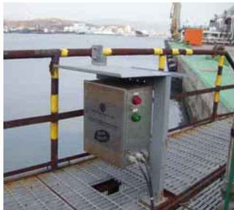
Figure 3B. Marine Terminal Pier-side/Wharf Installation.
