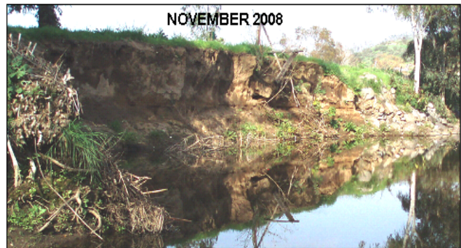
Bio-Engineering Stabilization of Severe Erosion On Escondido Creek, San Diego County
