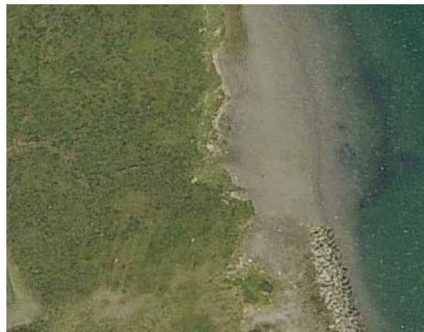
D-Street Marsh erosion along Sweetwater Channel
