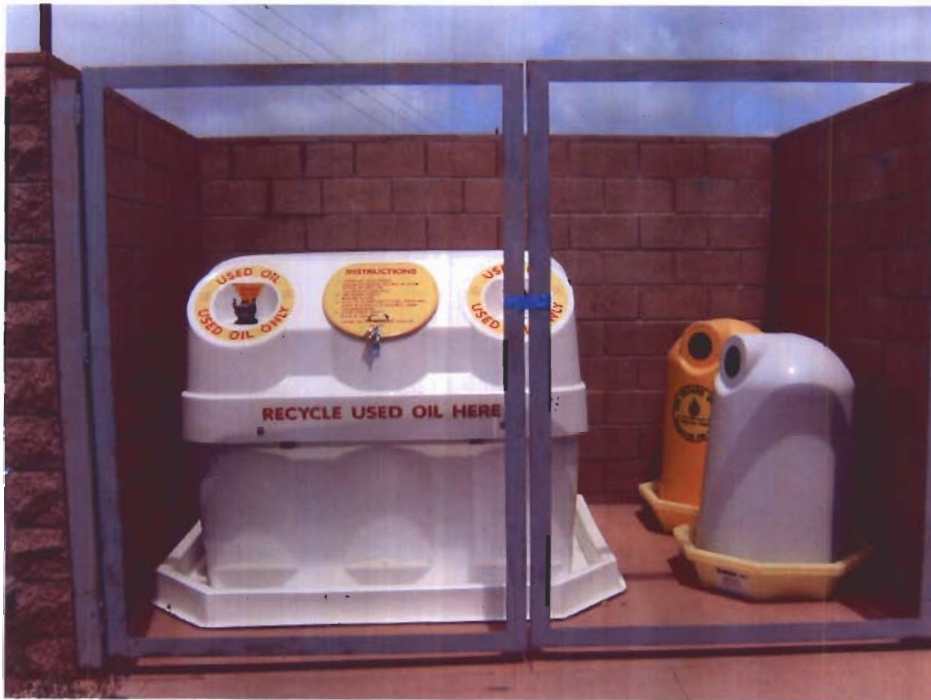
Photo #3 Used Oil Collection Center – awaiting construction of the roof
