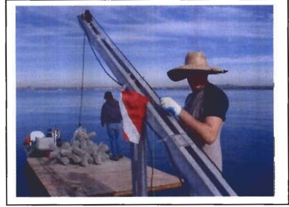
Photo 10. A-Jacks bundle being moved from transport vessel to placement vessel..
