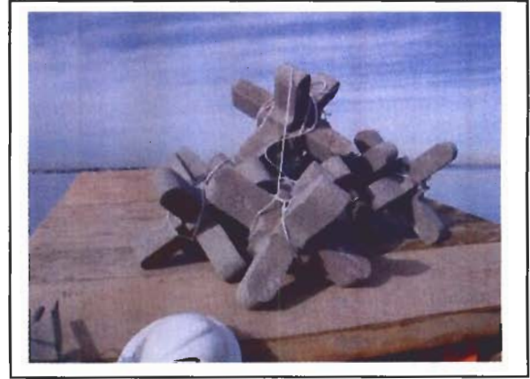
Photo 8. A-Jacks bundle on transport vessel being taken to placement vessel.
