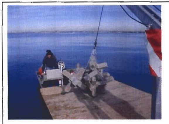
Photo 11. A-Jacks bundle being moved from transport vessel to placement vessel.
