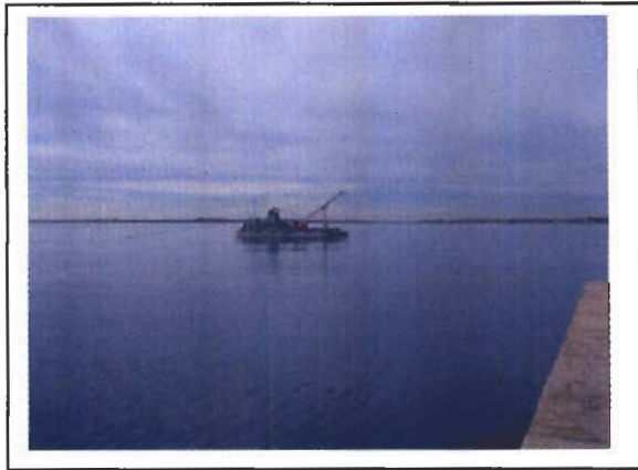
Photo 9. Placement vessel waiting to receive next bundle of A-Jacks.
