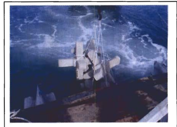
Photo 12. A-Jacks bundle being lowered into the water.
