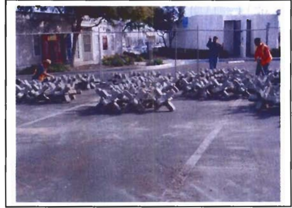
Photo 2. A-Jack reef components being assembled and bound.
