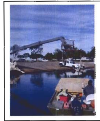
Photo 6. A-Jacks bundle being lowered onto transport vessel.
