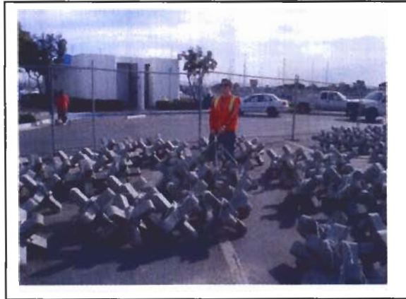
Photo 3. A-Jacks being bundled into groups of 8 components.
