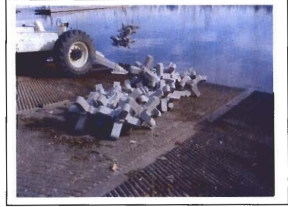
Photo 4. Bundles of A-Jacks waiting to be transferred to the transport vessel.
