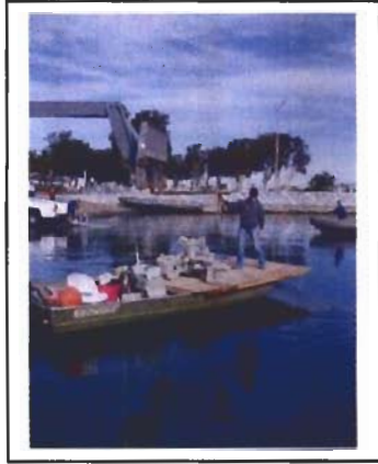
Photo 7. A-Jack bundle loaded onto transport vessel.
