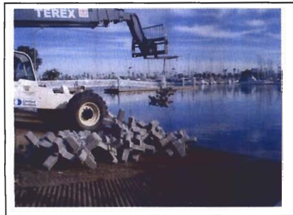
Photo 5. Bundle of A-Jacks being positioned for transfer to the transport vessel.
